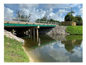
• Cypress Park Vehicular Bridge – Two lane, prestressed concrete pile supported bridge with rip-rap slope protection.
