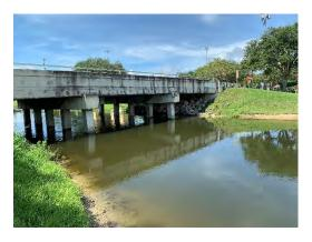
• Cypress Park Pedestrian Bridge – Pedestrian Bridge, likely supported on shallow foundations, protected by a concrete headwall.
