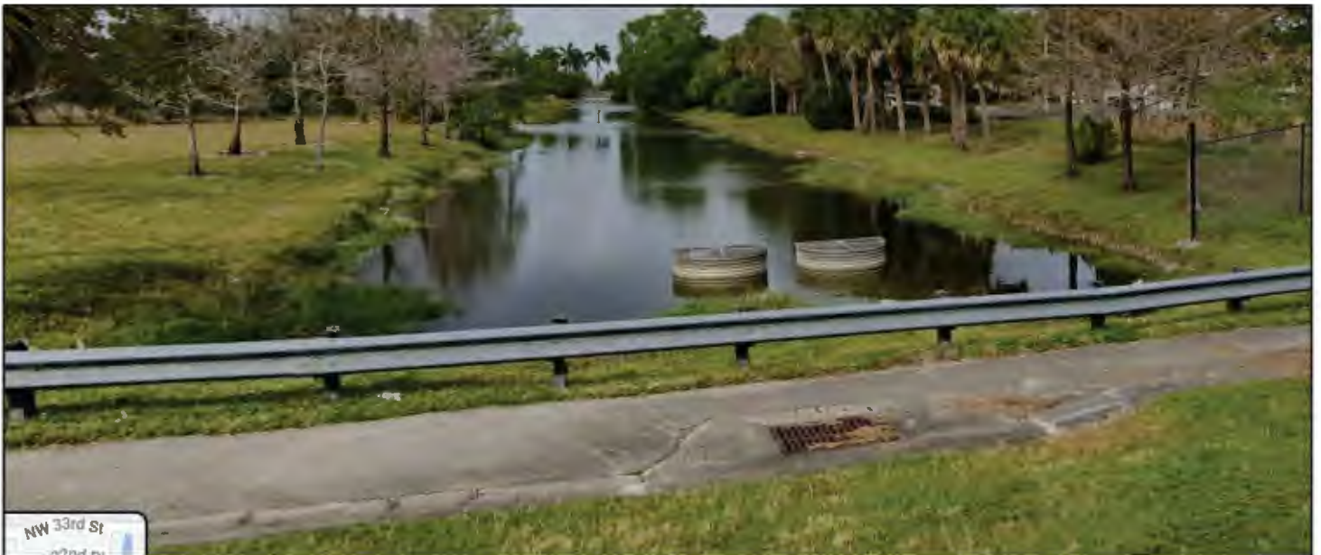
Figure 2 – Twin Risers Looking West from NW 123 rd Ave
