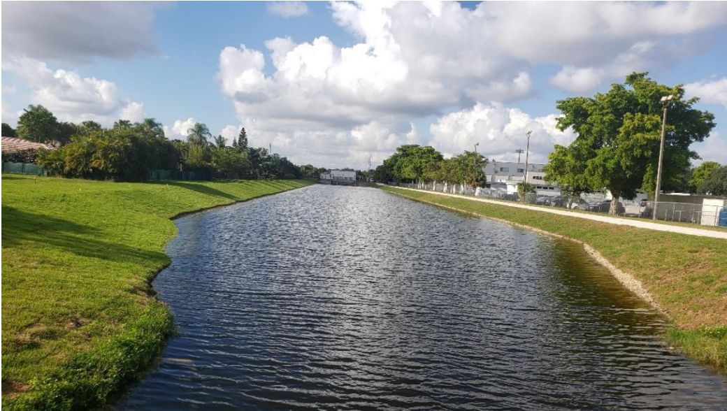
Photograph 1-Phase 2B Looking south from Riverside Drive 5.27.22 (Water Level = 7.2' NGVD)
