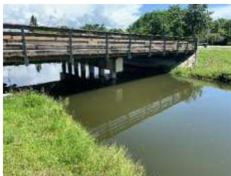
South Side of Bridge – View Looking North
