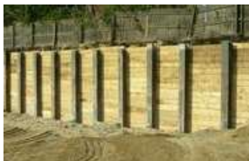
Example: H-Piles w/Lagging Boards
