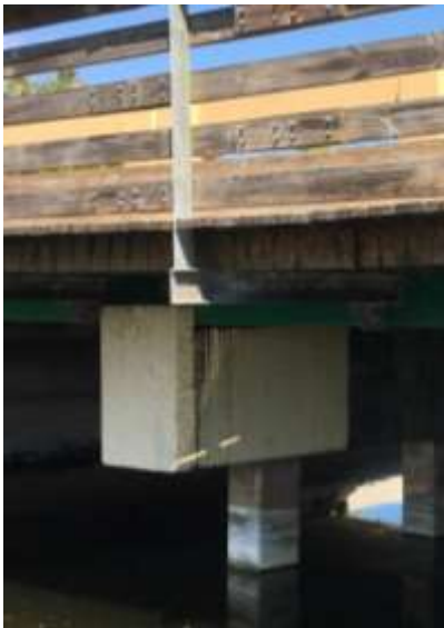
Added Sidewalk Extension
