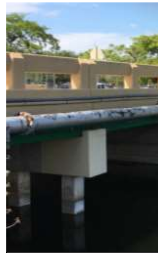
Added Pipe Support Extension
