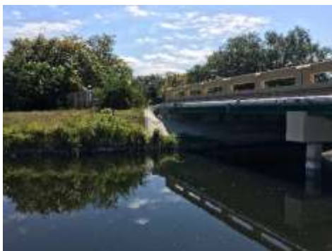
North Side of Bridge - View looking East
