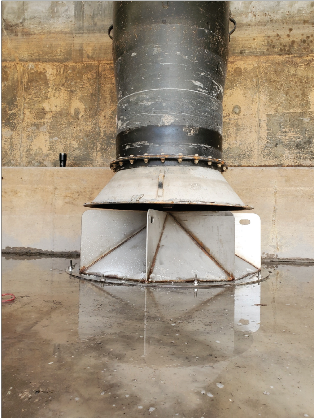
Figure 1-Vortex Suppression Cone
