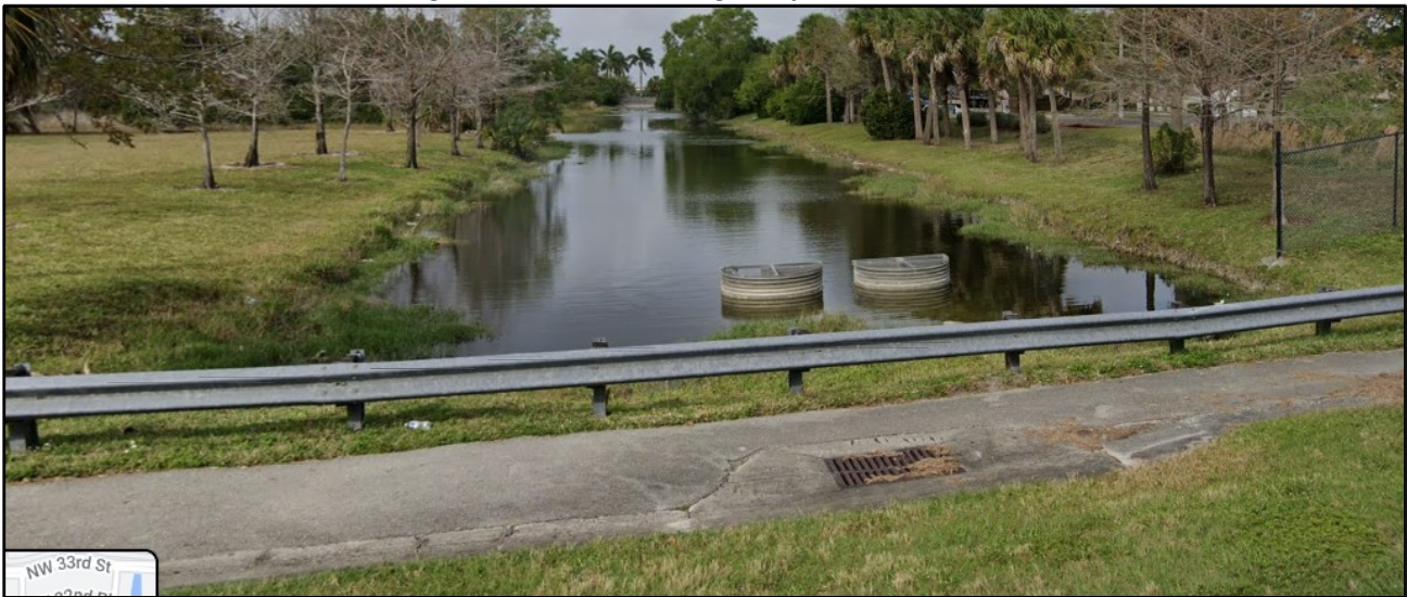
Figure 1 – Twin Risers Looking West from NW 123 rd Ave
